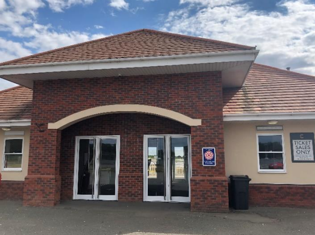
Entrance to Ticket Office
